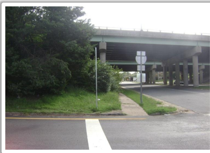
Photograph 7: Looking East from I-195 Off-Ramp Sight Distance Impacted by Vegetation
