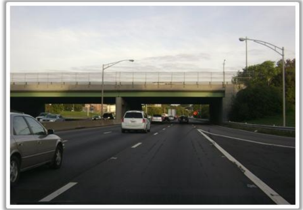
Photograph 5: Northbound I-95/I-64 Approaching the Belvidere Street On-Ramp
