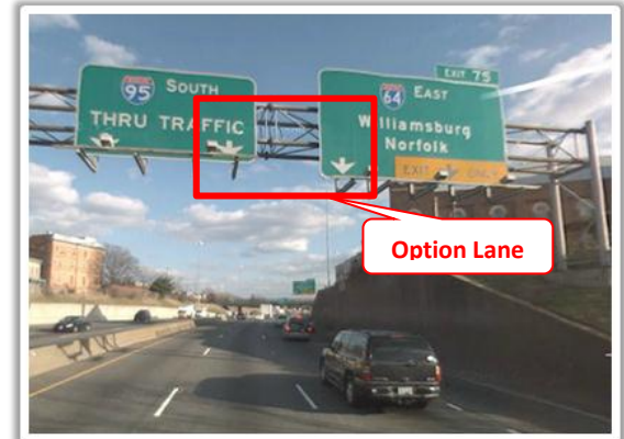
Photograph 12: Southbound I-95 to Eastbound I-64
