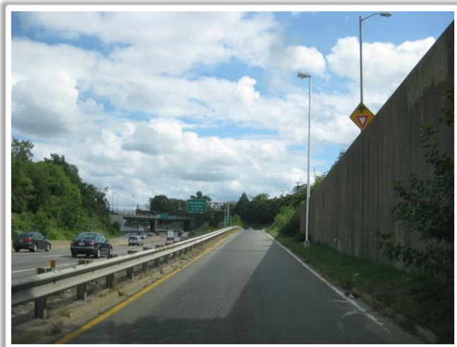
Photograph 2: Looking East from Collector-Distributor Road from Belvidere Street Loop On-Ramp
