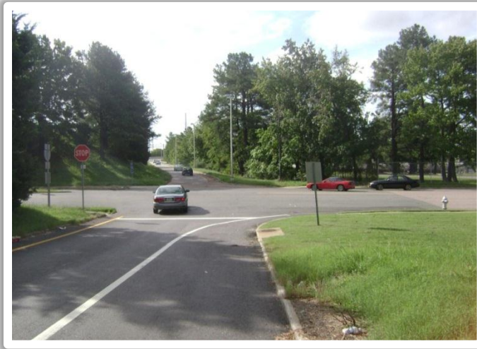
Photograph 6: Southbound I-195 Off-Ramp to Laburnum Avenue, Proposed Roundabout Location
