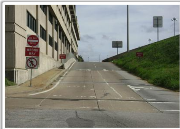
Photograph 11: Looking North at Southbound I-95 Off-Ramp to Franklin Street/15th Street
