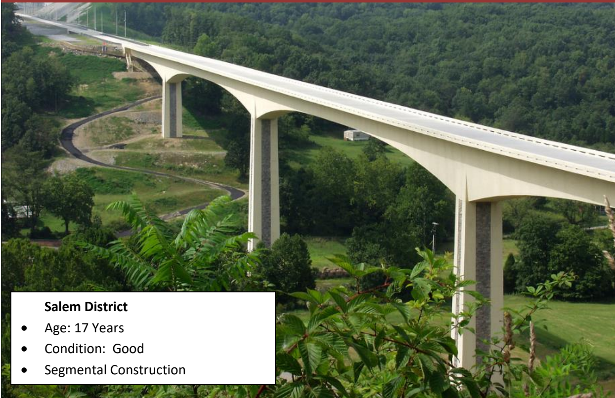
SMART Road Bridge (#17)
