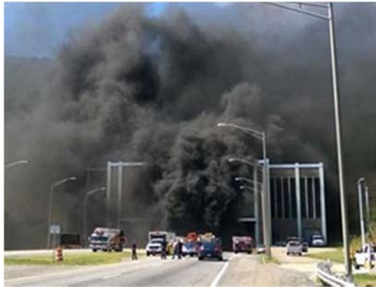
East River Tunnel Fire - July 2104
