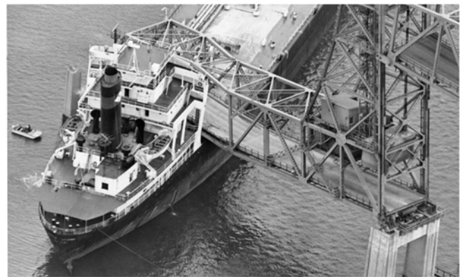
1977 Tanker Impact to Benjamin Harrison Bridge
