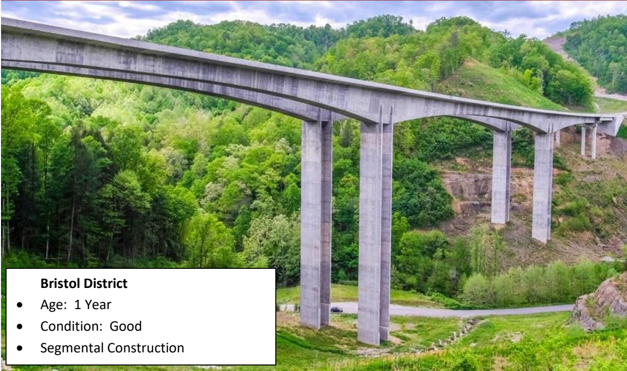
Route 460 over Grassy Creek (#16)
