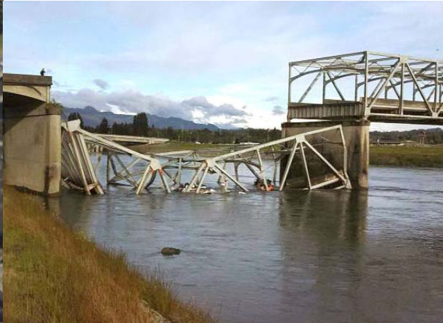
Skagit River Bridge
