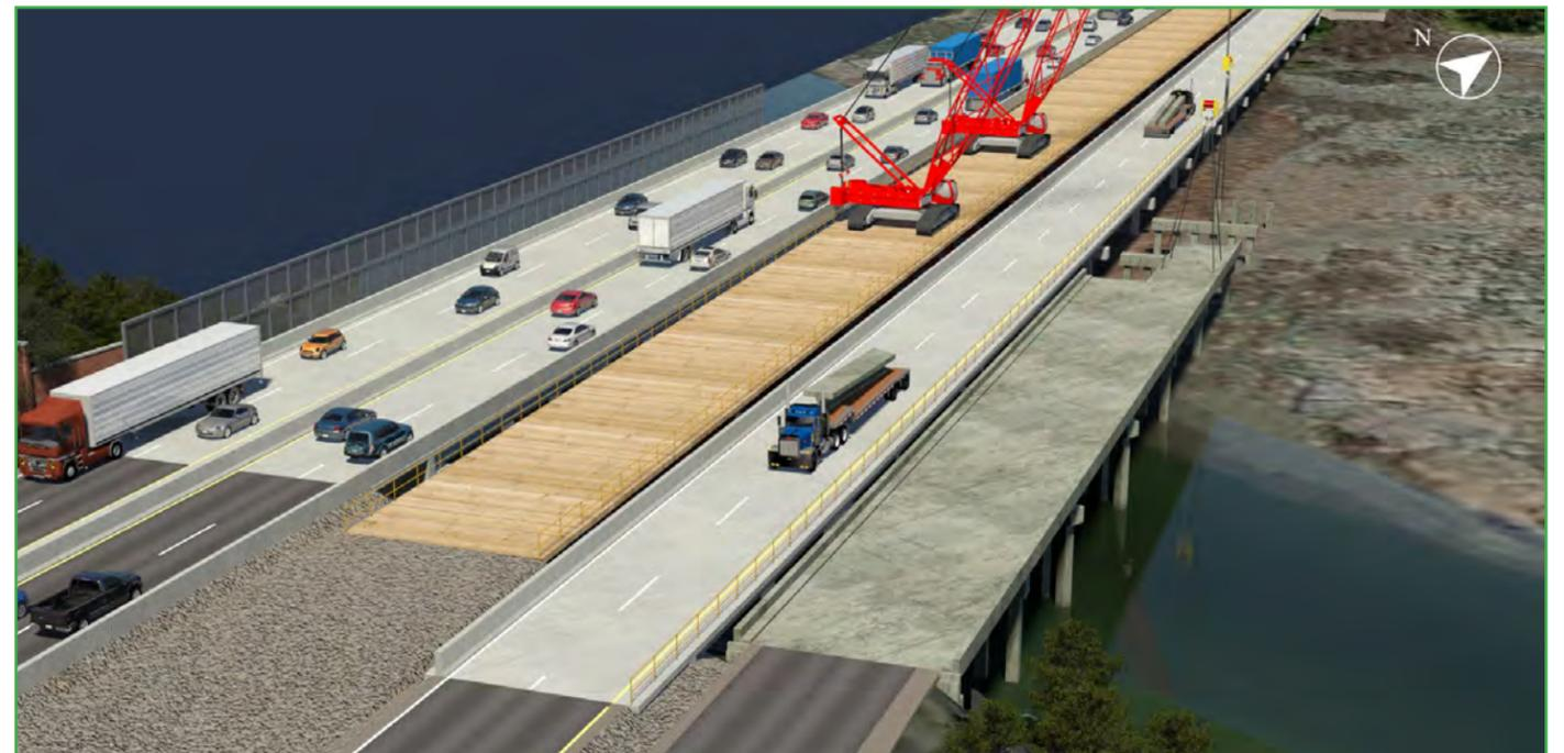
Figure 4.7.14: Demolish remainder of WB bridge.
