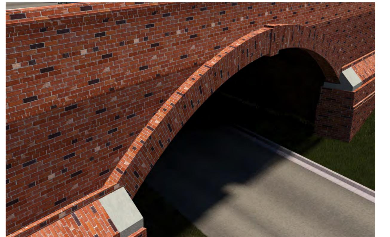
Figure 4.3.8: Colonial Parkway Aesthetics. Our design uses solid brick to blend the new portions of the widened arches with the existing arches.
