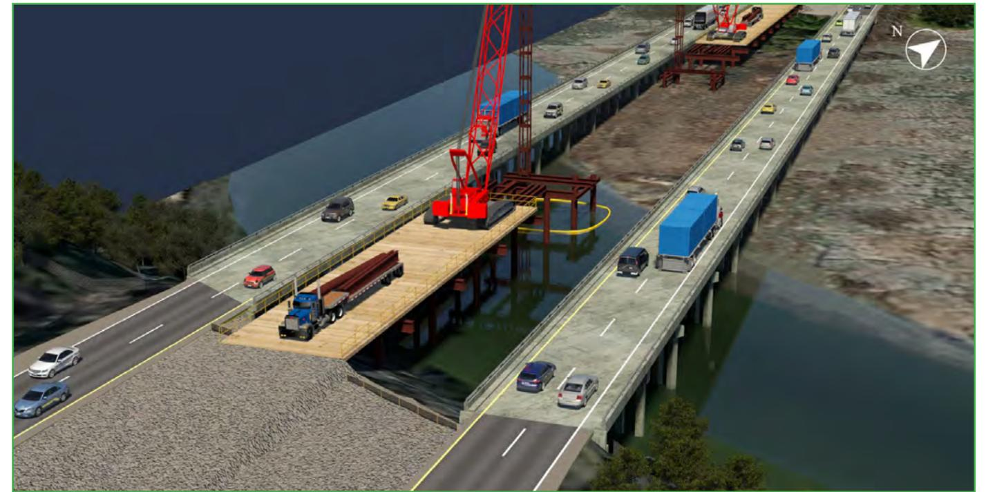
Figure 4.7.4: Construction of 40 foot span construction access trestles. Piles to be installed prior to the beginning of the February Anadromous fish window.
