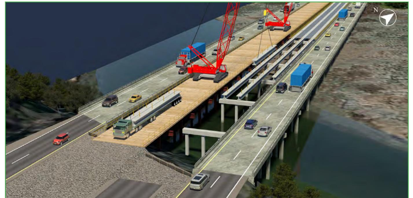
Figure 4.7.6: Install superstructure items with access and material lay down areas in the I-64 median at both ends of the bridge.
