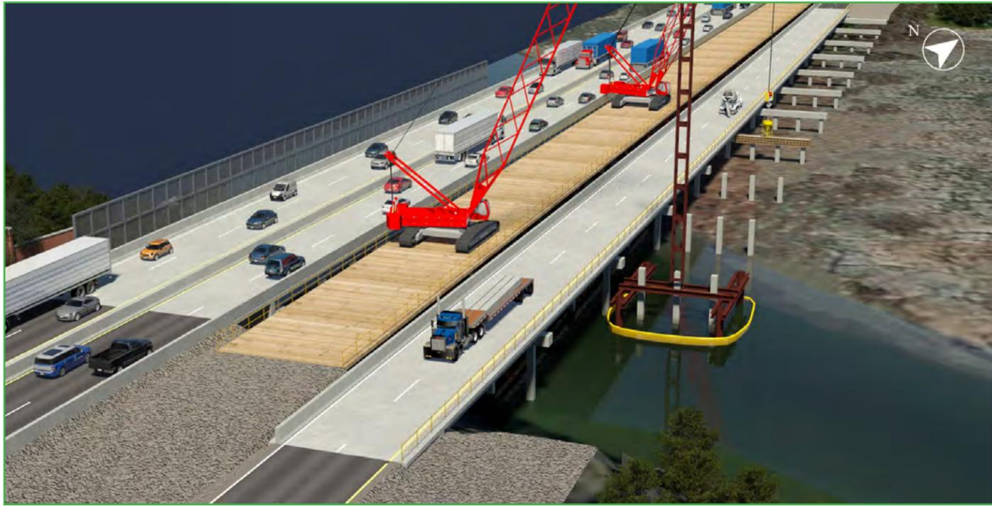
Figure 4.7.15: Install substructure.
