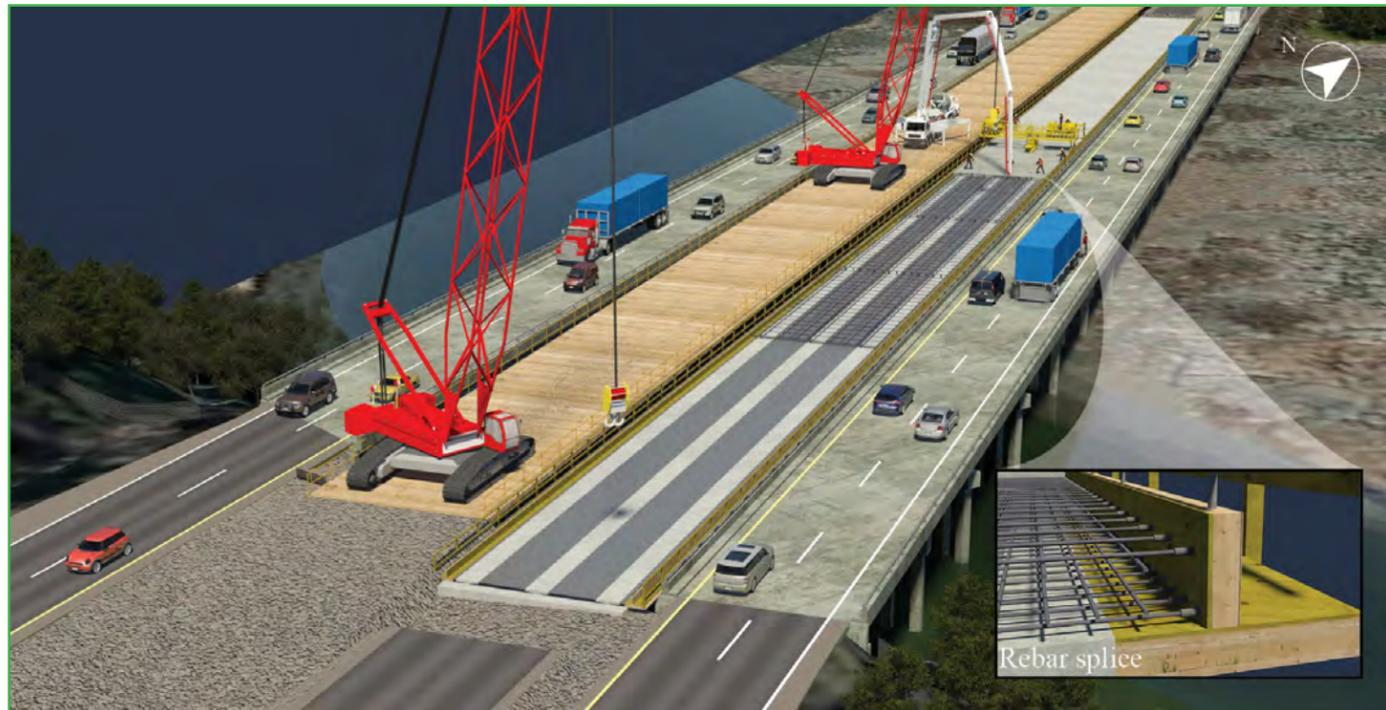
Figure 4.7.7: Install stay in place deck forms stainless deck reinforcing steel (rebar splice detail shown for construction of WB widening in Phase 3).
