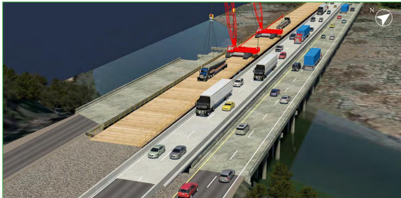
Figure 4.7.9: Phase 2 - Demolish existing EB bridge.
