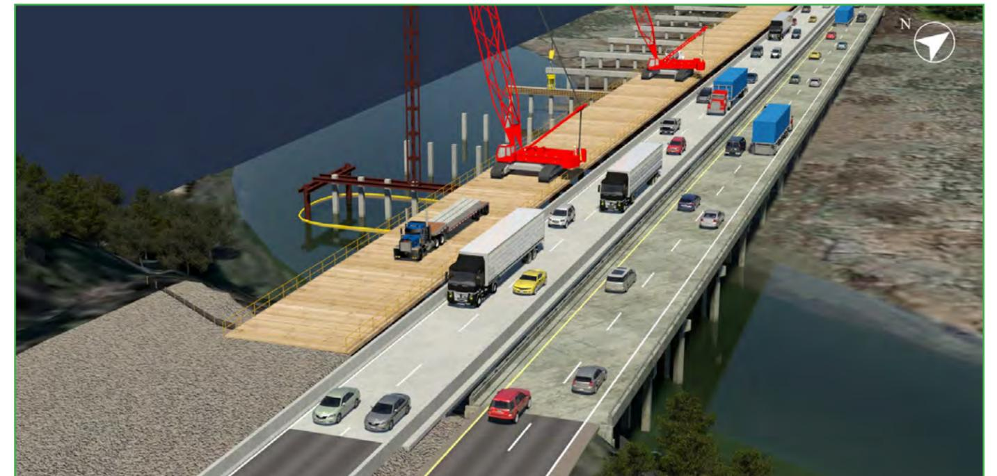
Figure 4.7.10: Install substructure.
