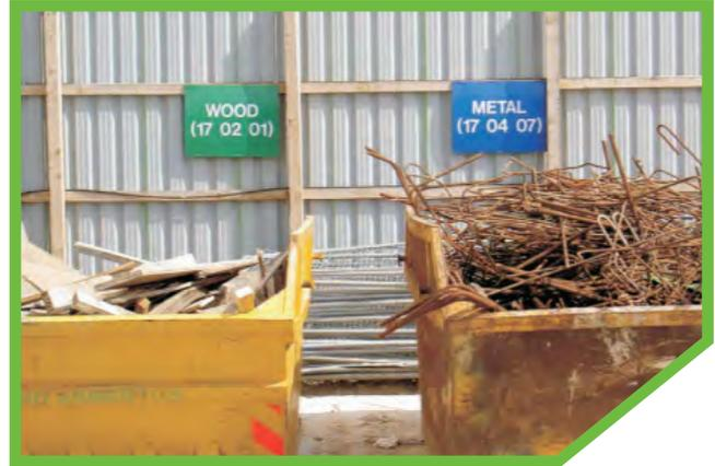
**Figure 4.5.15: Segregating Recyclable Materials.** We place containers and signs to segregate waste, which encourages and streamlines recycling and re-use.
