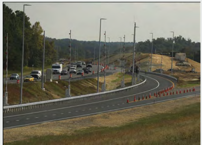
Figure 5: VDOT I-95 Southern Terminus Extension
