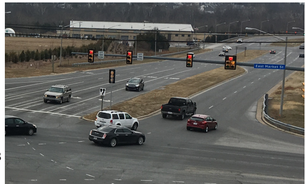
Potential Conflicting Transmission Lines at Route 7 and Battlefield Parkway
