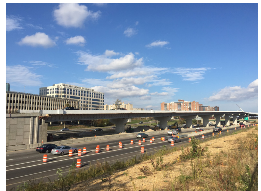
Implementation of TTCP on I-395 HOV Ramp at Seminary Rd.
